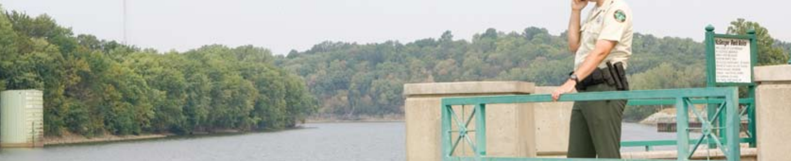
Odom at the dam where the accident occurred.
